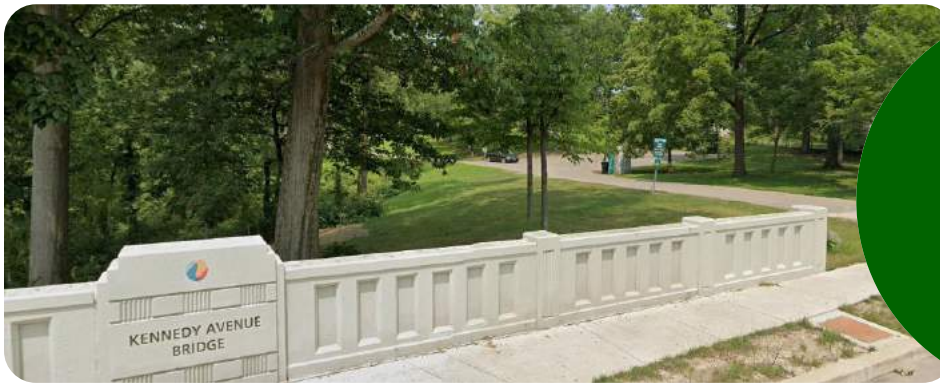
Kennedy Avenue Bridge & Kennedy Heights Park
